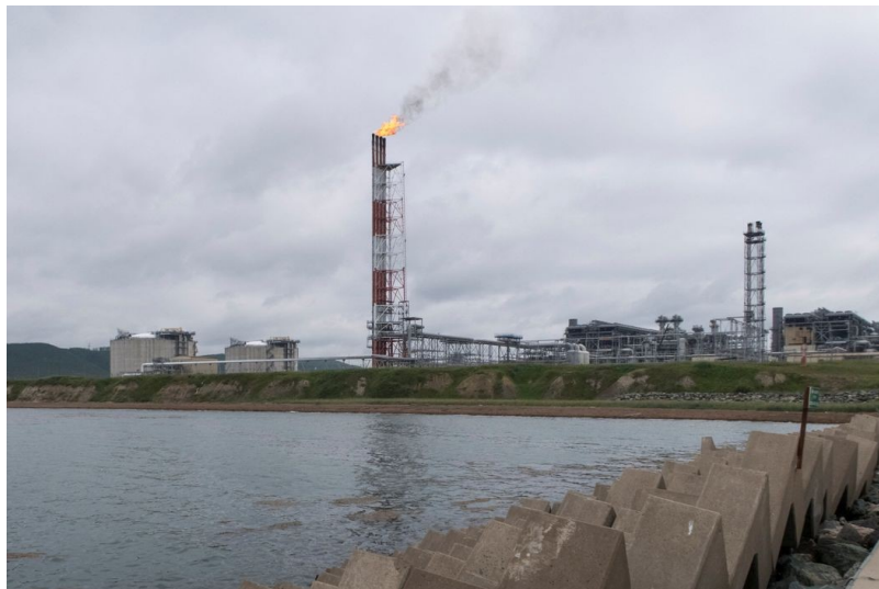
A natural-gas plant on the Russian island of Sakhalin.
