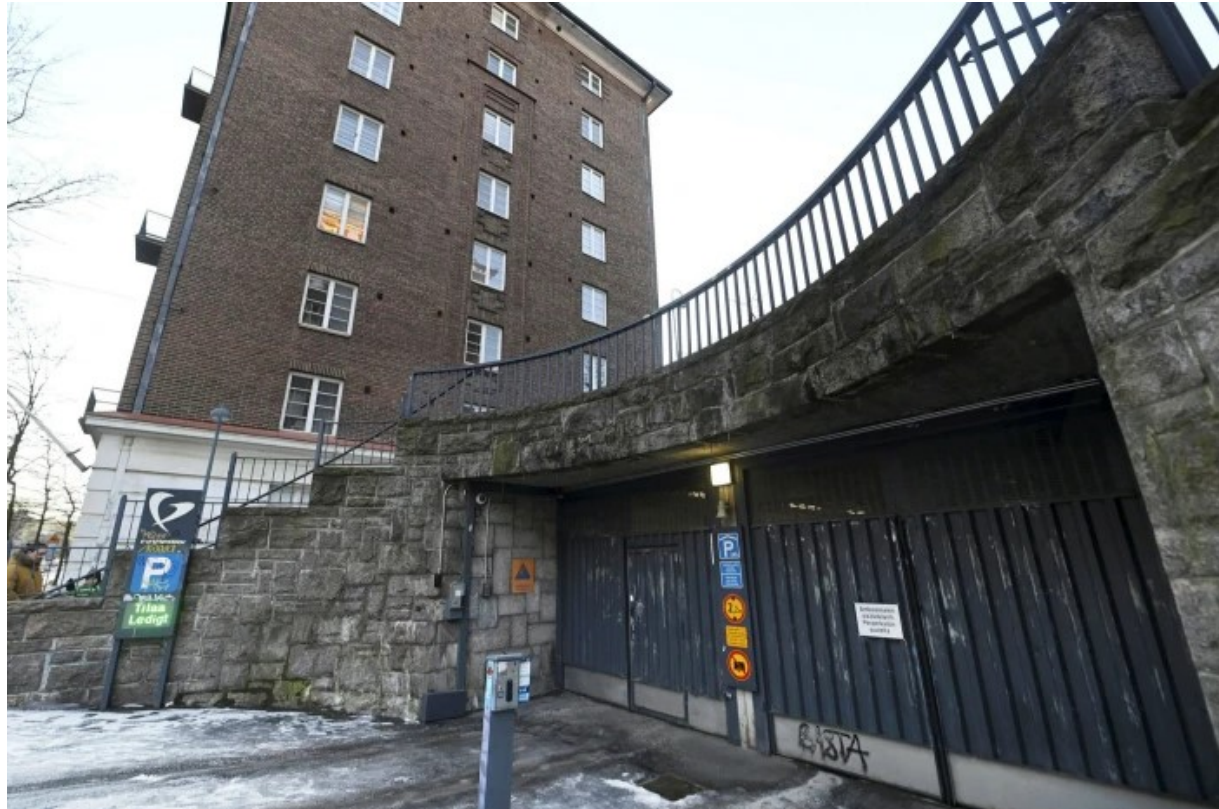
An emergency shelter in Kallio, Helsinki. All buildings above a certain size have to have their own bomb shelters © Lehtikuva
