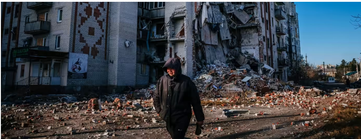
A damaged residential building in the city of Lyman, Donetsk region. War in Ukraine underscored the danger of leaving states in a geopolitical 'grey zone', outside both Russia and western spheres © AFP via Getty Images
