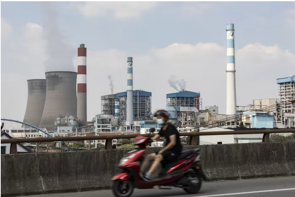
A power station in Jiangsu. China's provinces have accelerated approvals of coal-fired power plants © Qilai Shen/Bloomberg
