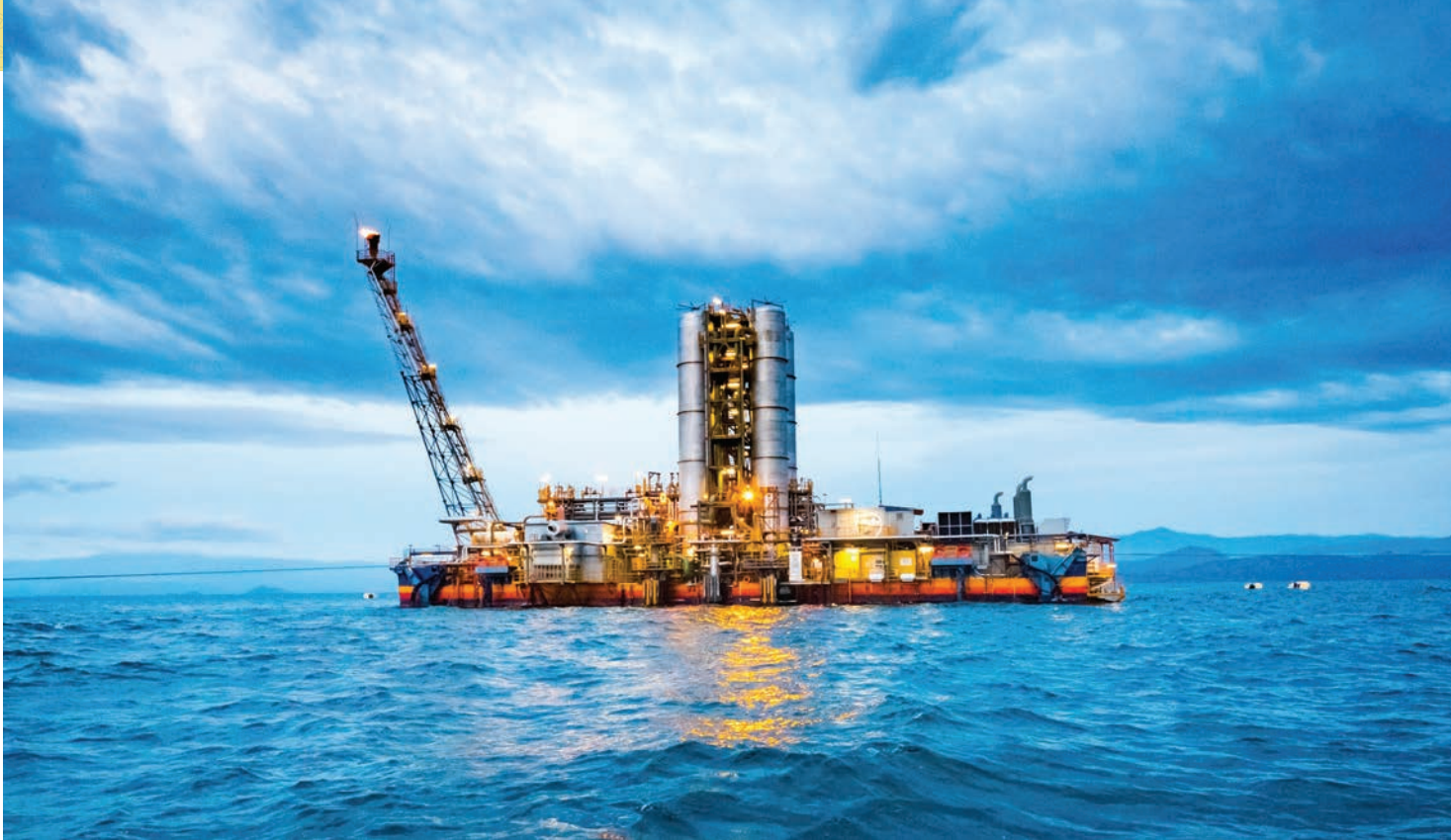
The KivuWatt power project in Rwanda is unusual and important ecologically.
