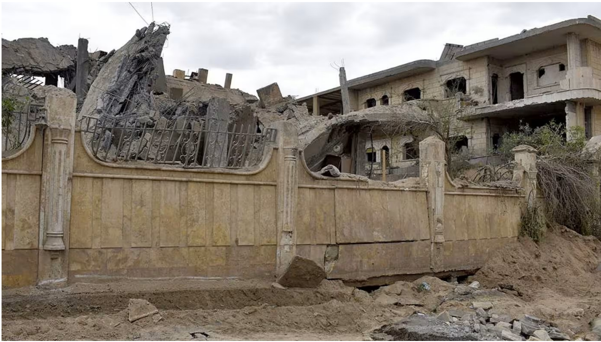
A damaged building following an air strike in Syria's Deir Ezzor on March 26. Local media said at least 15 people were killed in the attack © AFP/Getty Images
