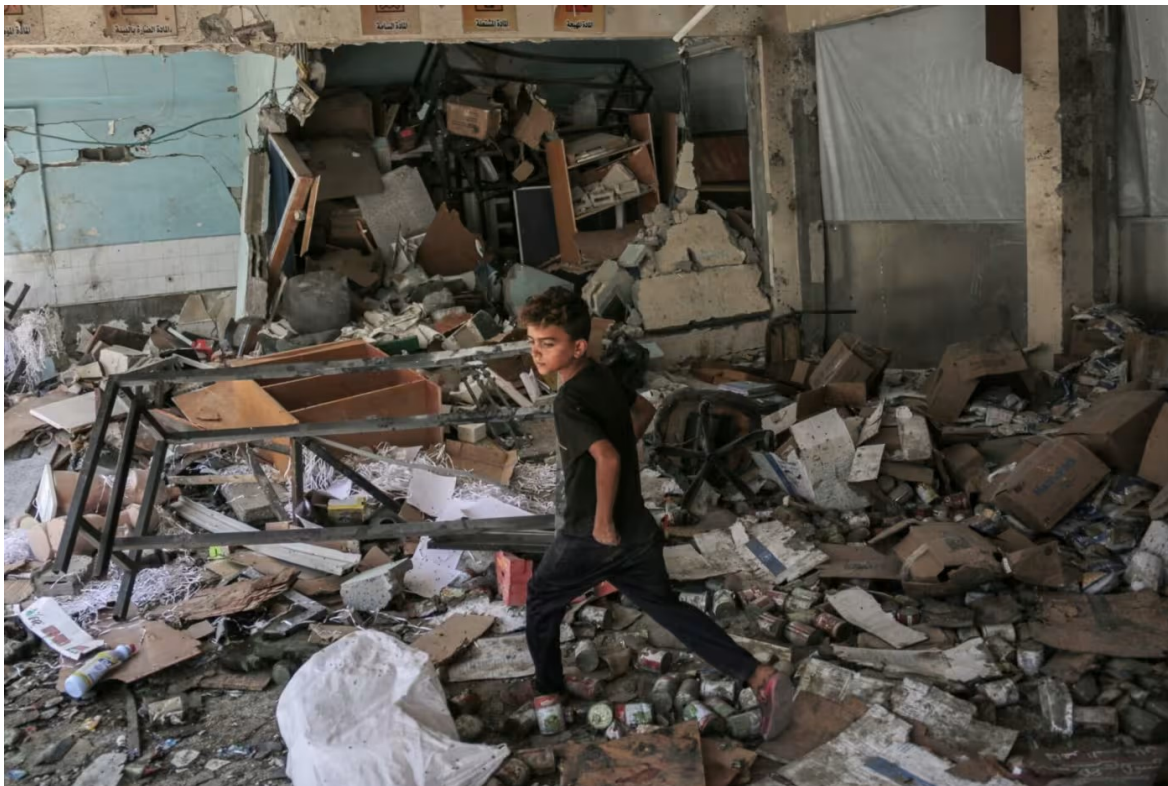
Inside the heavily damaged al-Jaouni school © Ahmad Salem/Bloomberg
