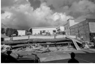
Rescuers are seen at the site of a collapsed building after a powerful earthquake struck Port Vila, the capital city of Vanuatu, on December 17. Photo: AFP
